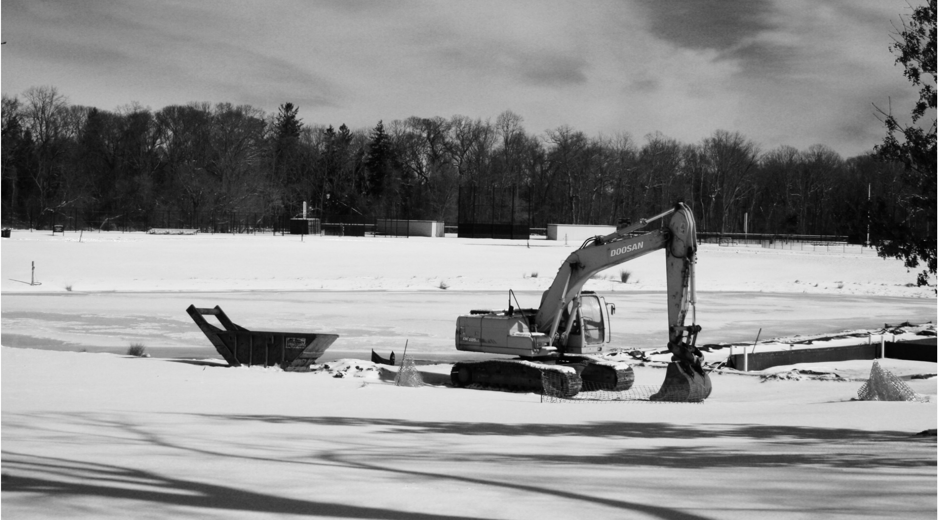
The construction project in front of the Wellness Center has been going on since this past summer.
